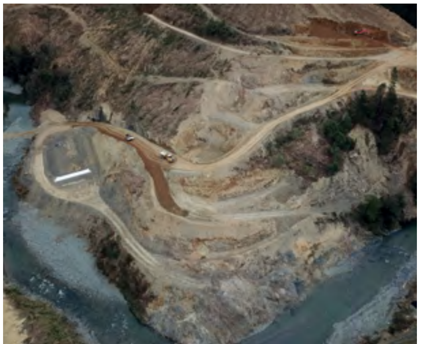
Careful construction – preparing the right-hand side of the dam.
