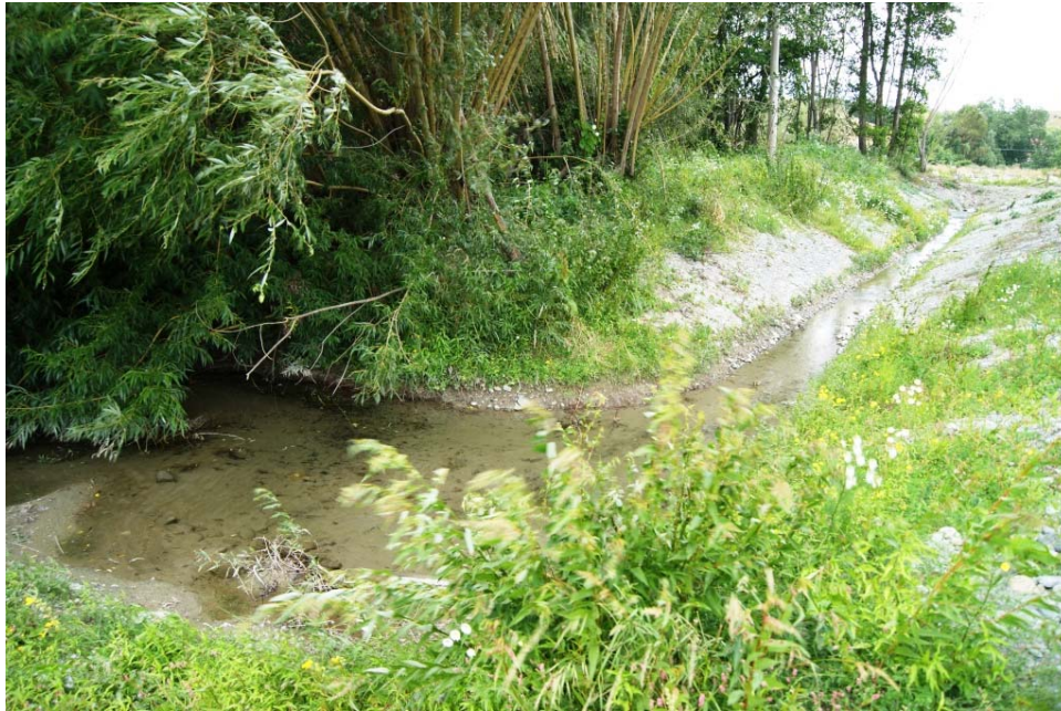
Figure 4-1: The bypass channel near the Opihi River. Near the river the bypass channel becomes wide and shallow as it disperses amongst willows and scrub.
