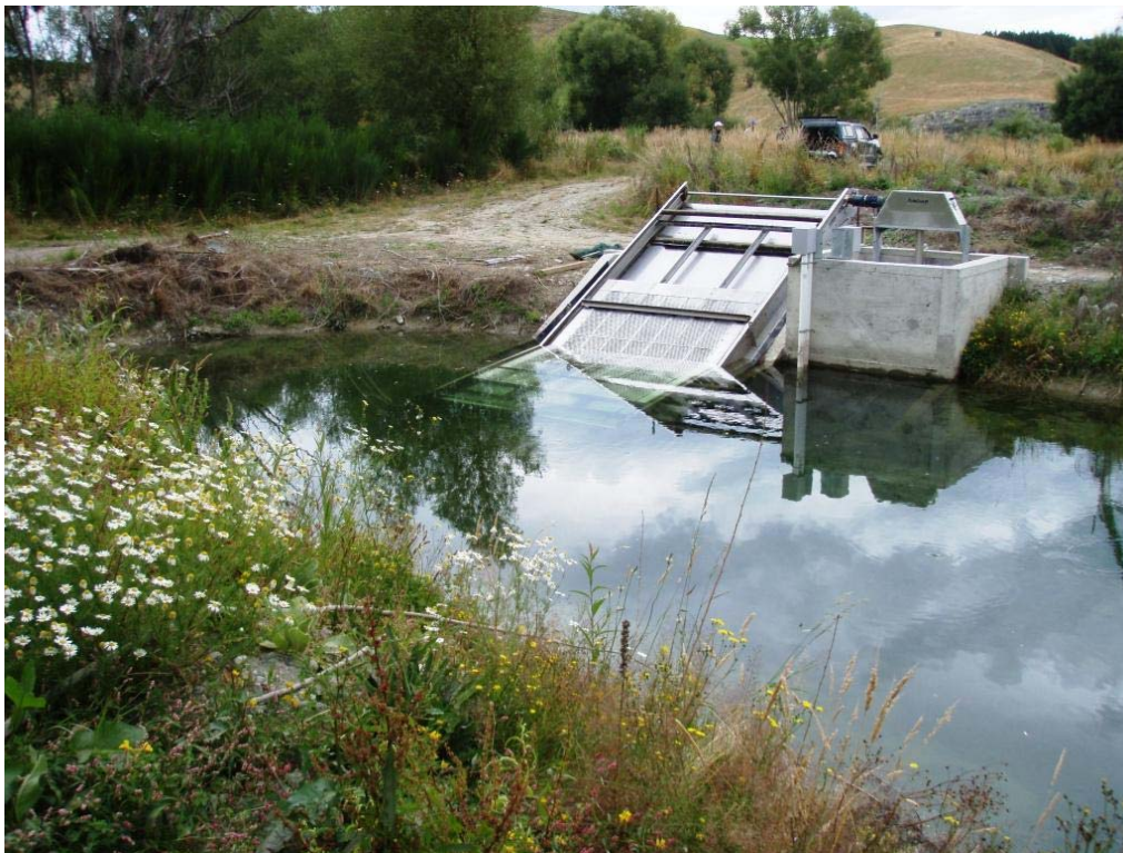
Figure 2-3: The Andar screen and intake pond on the Totara Valley scheme. Water flows from the pond, through the screen and down into a channel behind the screen (adjacent to the parked vehicle).
