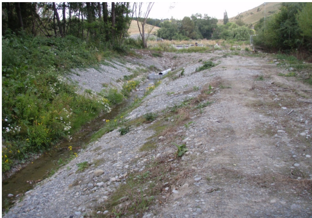
Figure 2-7: The bypass channel. Water from the outlet pipe flows along the bypass channel and back to the Opihi River.
