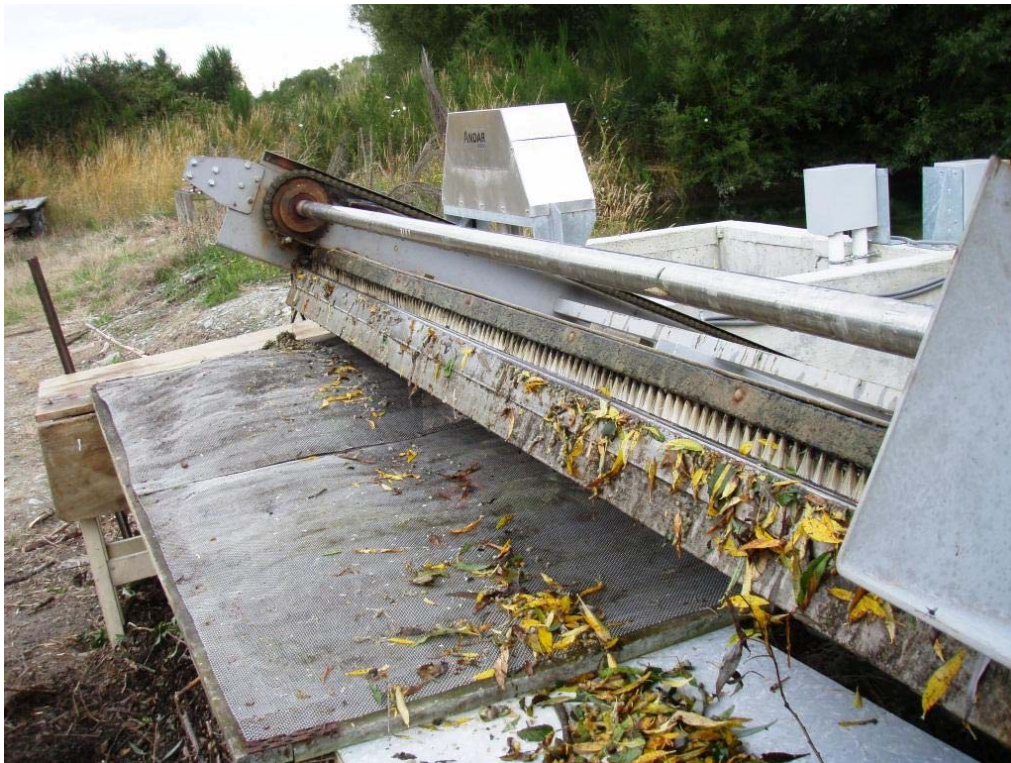
Figure 2-4: The outer coarse screen, and (at left) the inner fine screen. Screens are cleaned by constantly moving brushes as at right of picture, and by rubber squeegees.
