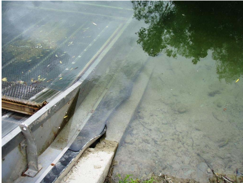
Figure 3-3: The rubber flange on the Andar screen. The black rubber flange appeared to be fitting poorly to the concrete base; in the foreground a gap between the concrete and flange can be seen. This gap is mostly out of the water and consequently has little effect on fish - however any such gaps in deeper water might allow a strong flow of water that bypasses the screen, and draw fish through directly into the scheme channel.
