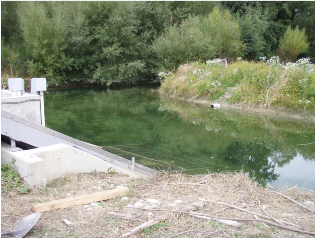
Figure 2-6: The bypass pipe. On the northern bank of the pond - opposite the screen - is an outlet pipe leading to the bypass channel.
