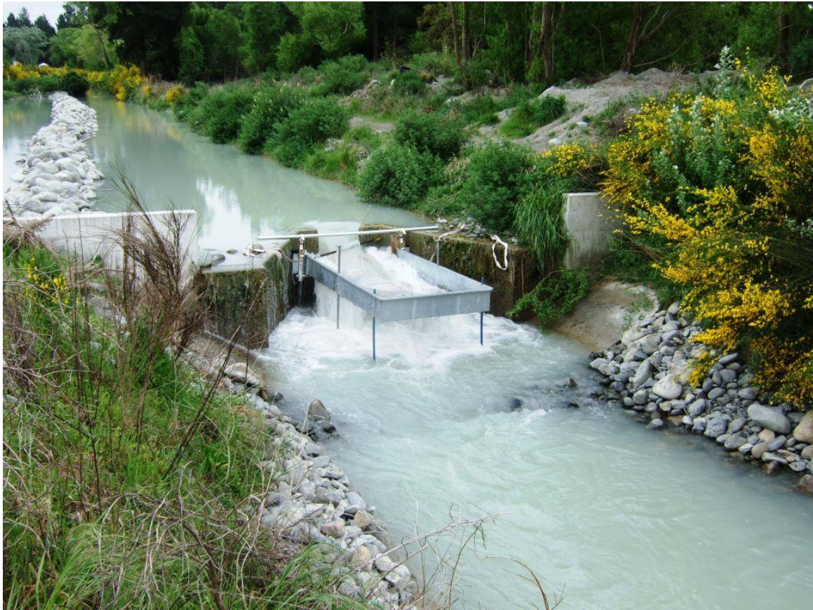
Figure 2-4: The fish trap on the bypass channel. The permeable rock bund can be seen in the background, and upstream of the trap.
