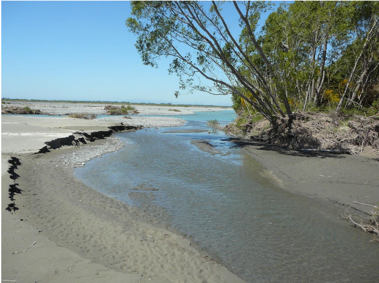
Figure 4-1: Bypass channel returning water to a braid of the Rakaia River, c. 1.4 km from the Acton intake. Note that the flow in the channel here is greatly reduced from the 1.0 \text{ m}^3\text{sec}^{-1} bypass flow requirement.
