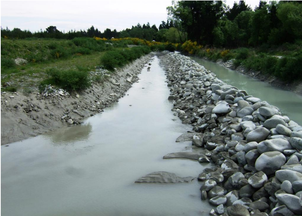
Figure 2-2: The permeable rock bund at the Acton intake, photographed looking upstream and with low water levels. The diversion channel supplying water can be seen the right of the photograph, and the scheme intake channel to the left.
