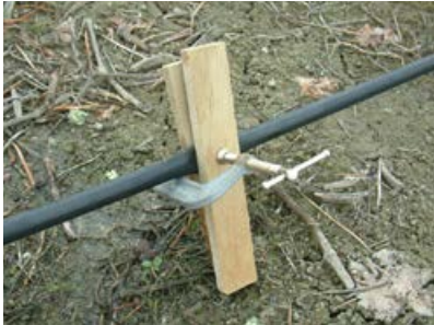
Figure 1. Clamping lateral to reduce in-line pressure.
