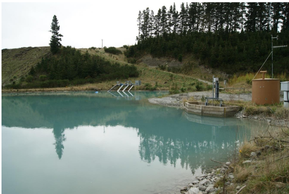
Figure 2-4: The headpond as seen from near the bypass weir. In the foreground the SDC intake control (brown cylinder) and headworks for the infiltration galleries (bunded structure). The galleries are underwater and under a layer of gravel and boulders in the centre foreground of the picture.
