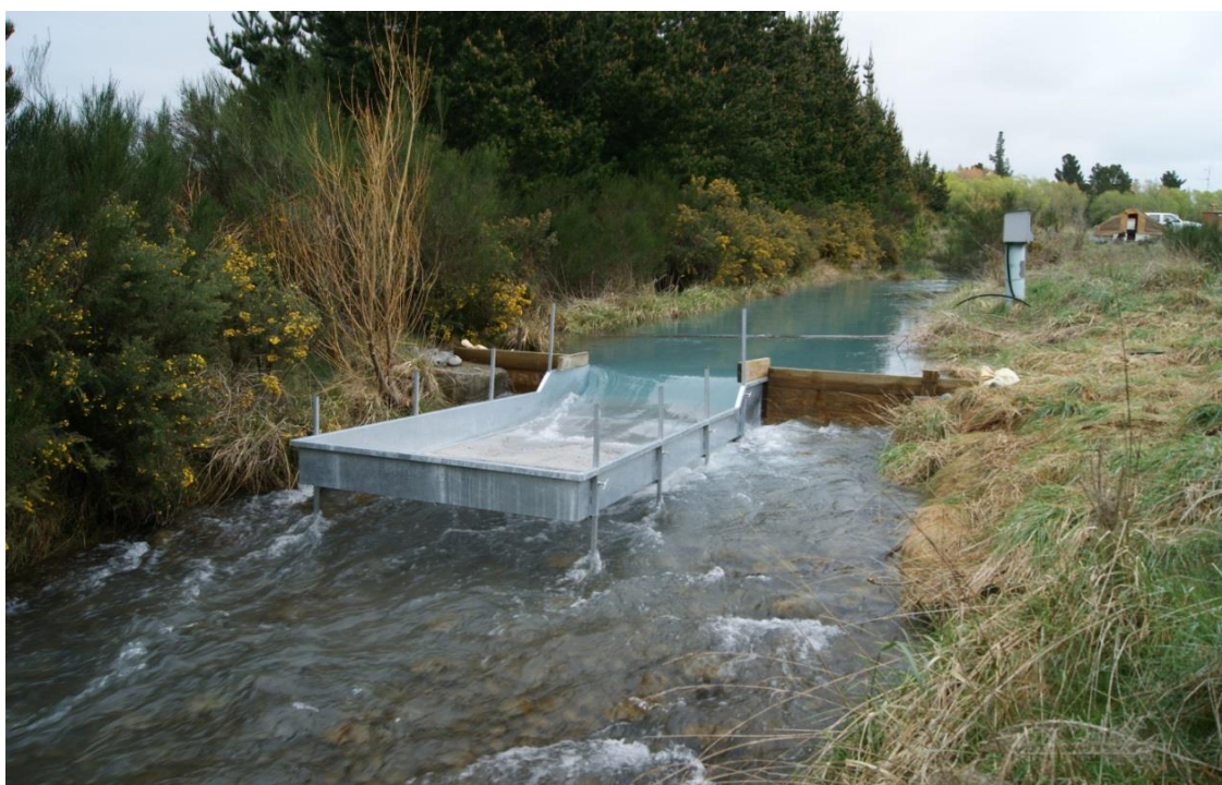
Figure 2-5: The intake trap. Water passing through the infiltration gallery flowed into the scheme intake channel and then through the trap.
