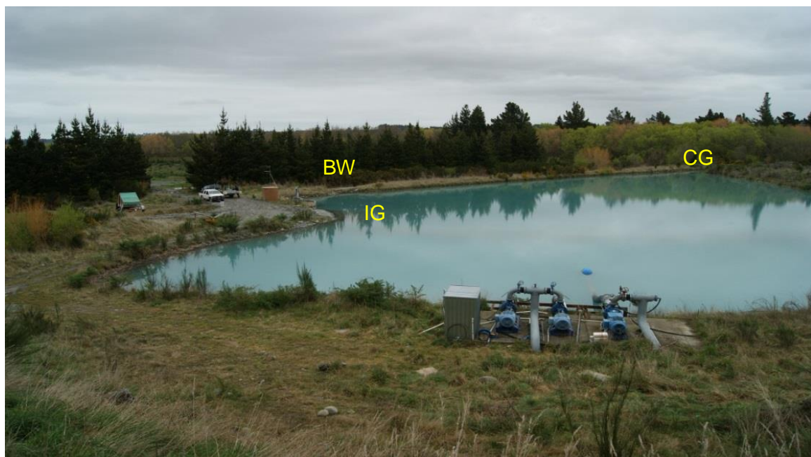
Figure 2-2: The headpond. The infiltration galleries (IG) and SDC intake are situated near the vehicle seen on the left, and the bypass weir (BW) is just visible on the edge of the pond to the right of the vehicle. In the foreground are the pumps for the Grasslands intake (not operating during this trial), and on the far right of the headpond is the control gate (CG) for water entering from the Rakaia River via the inlet channel.
