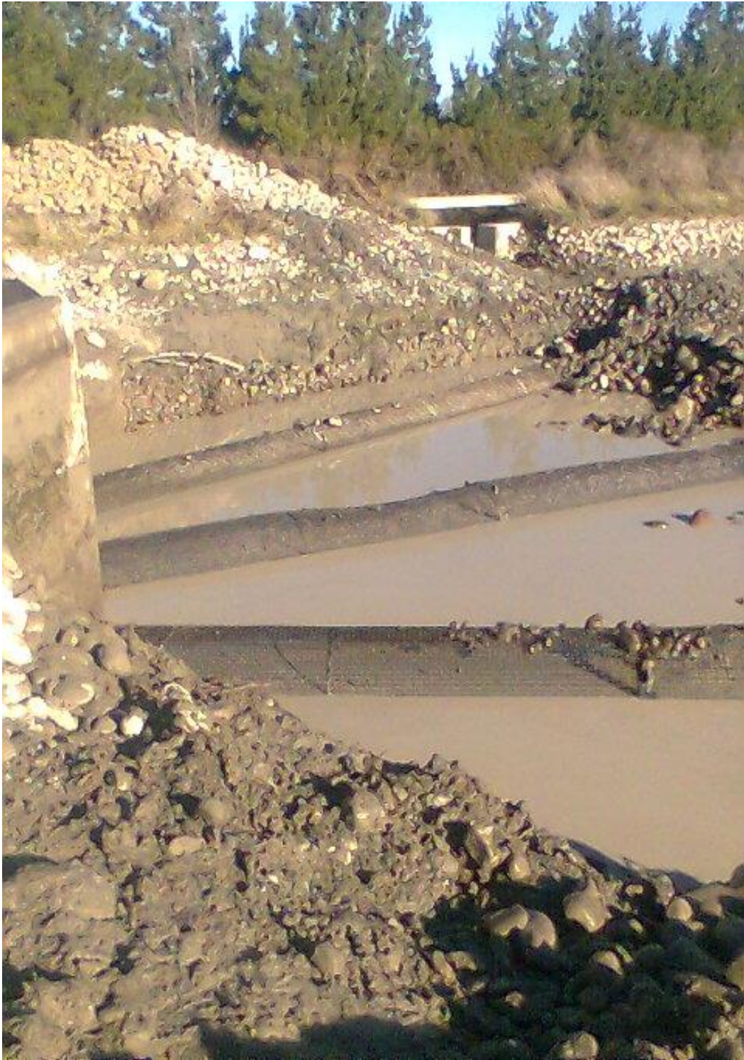
Figure 2-3: The infiltration gallery pipes, Winter 2012. Screen material and silt had been removed during maintenance and new material was replaced before the headpond was refilled.
