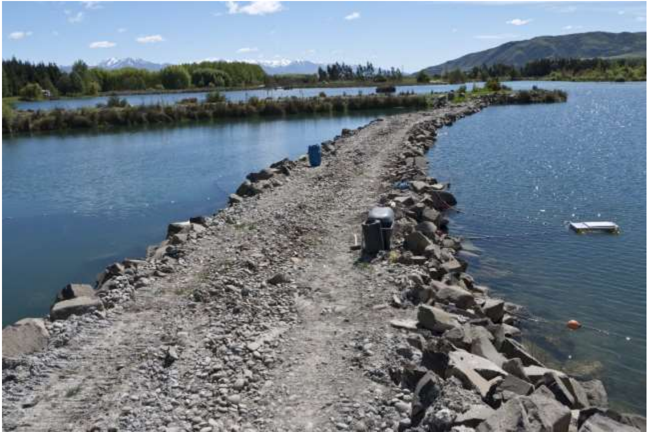
Figure 3-2: The NOIC bund. Dye marked salmon were placed in the enclosure seen to the right of the bund; any fish that passed through the bund was collected from nets placed downstream, seen on the left.
