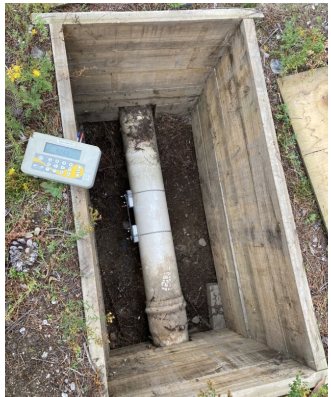
Image: A clamp-on ultrasonic meter is installed on the length of pipe, the transducers are strapped onto the pipe at a spacing determined by the meter after considering the installation parameters.
