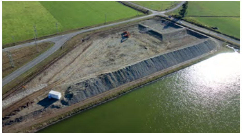
A pilot managed aquifer recharge project in Mid Canterbury is raising groundwater levels and reducing nitrates.
