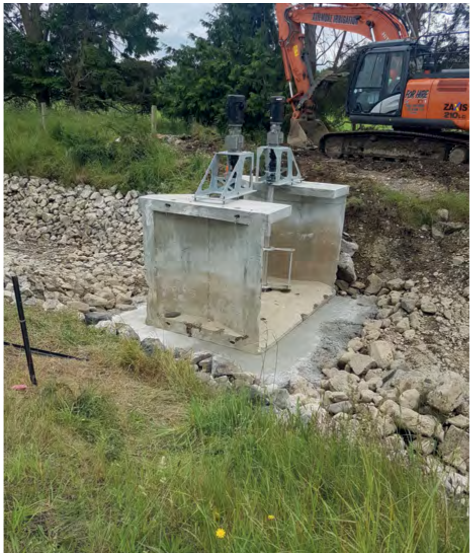
Turbines during installation.
