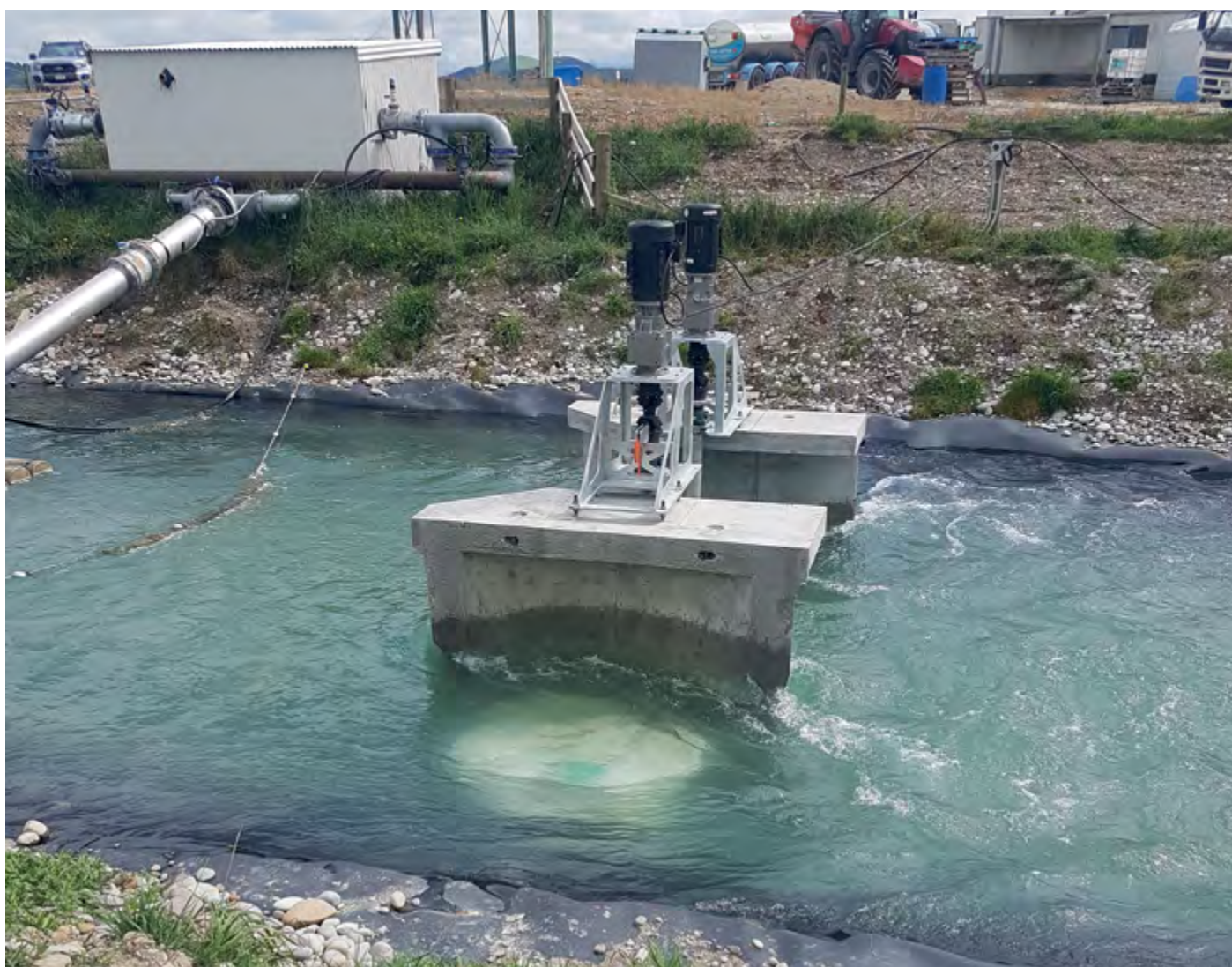
Twin turbines installed in the main race at Rotoma Farm.
