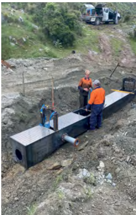
The Bossman screen being settled into the channel.
