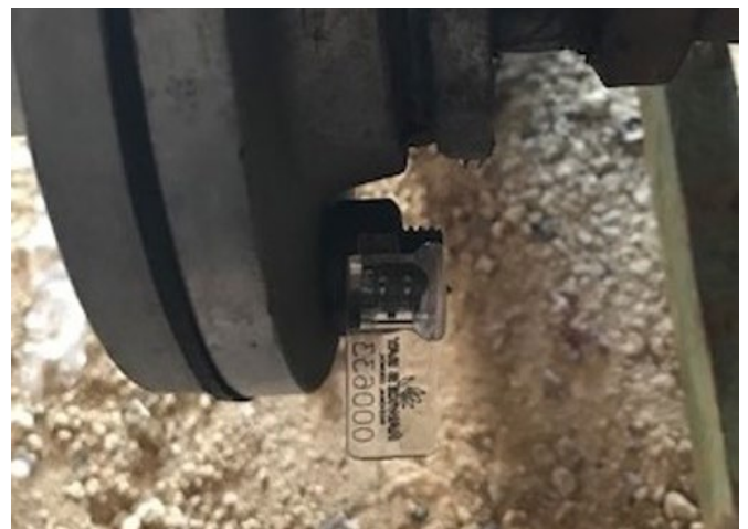
Image: An example of a Tamper Tag with a unique serial number inserted onto a bolt securing a flange.
