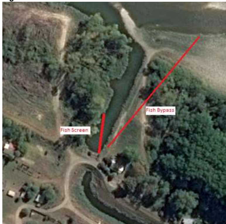
Figure 4: Before Debris Screen
