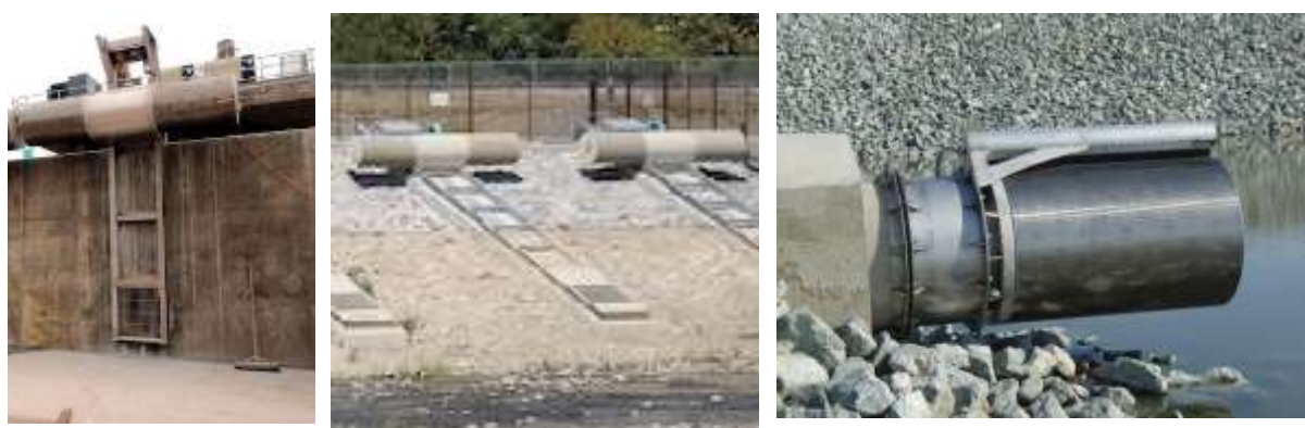
Figure 10: Cylinder screen construction types
