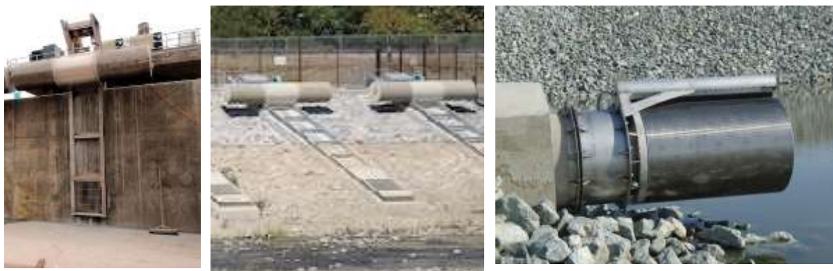
Figure 7: Cylinder screen construction types
