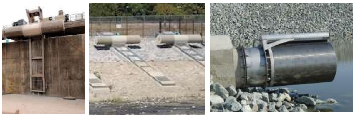
Figure 11: Cylinder screen construction types
