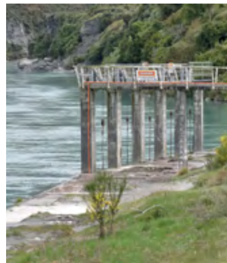
Left: The RDR intake structure at the flood peak. The walkway structure is normally 4.5m above the river level (see picture above).
