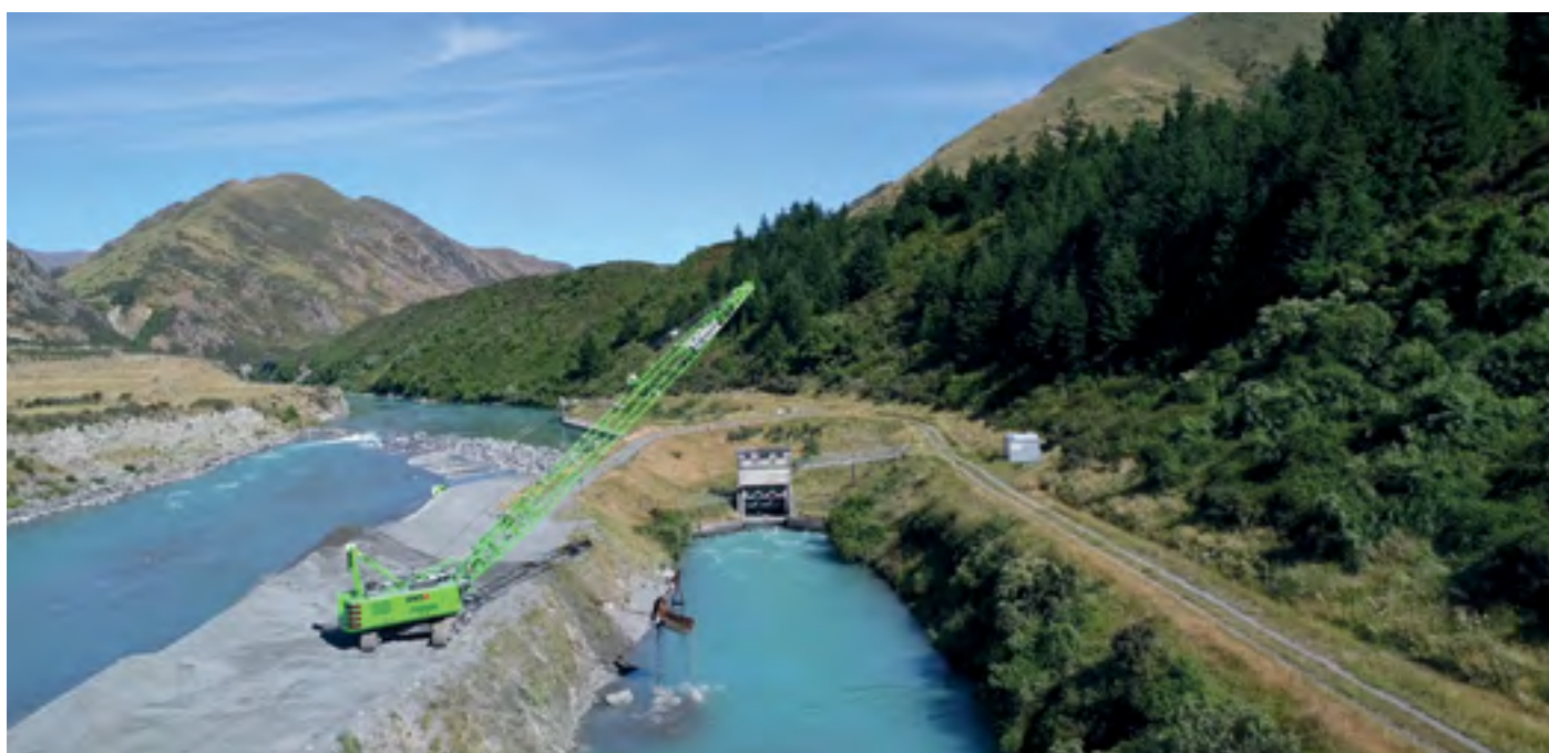
The dragline (crane) operating at the RDR intake canal to remove deposited gravel and sand following a high flow event. The in-river control weir is evident just upstream with the intake structure partly obscured behind the dragline boom.
