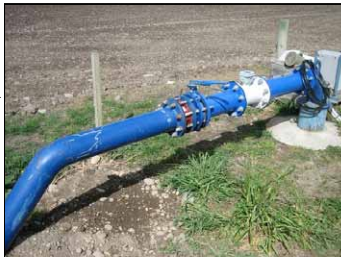
SeaMetrics electromagnetic meter – internationally tested and Environment Canterbury compliant
