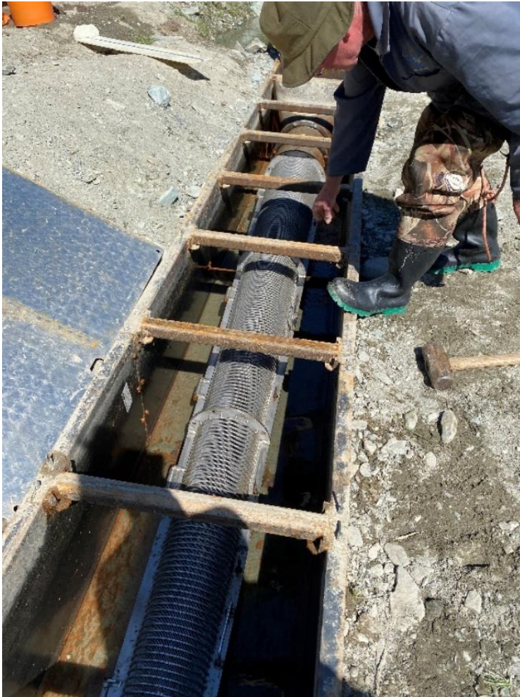
Photo 3. Upstream internal view of fish screen with covers off, December 2021.
