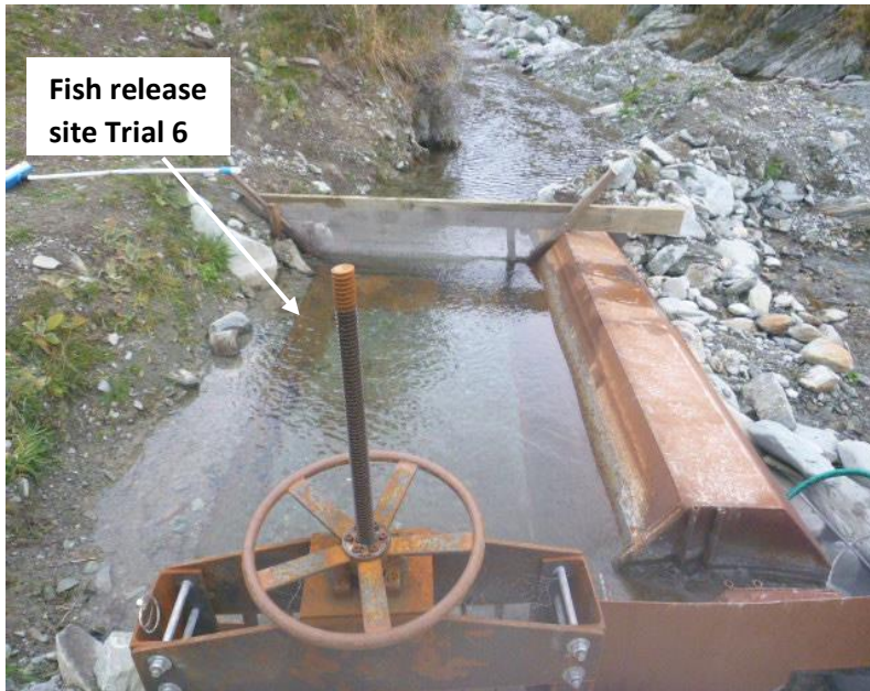
Figure 6 Screen intake and control gate (foreground), prefabricated steel apron insert, fitted upstream fish proof barrier and upstream fish bypass (lower right). June 2022.
