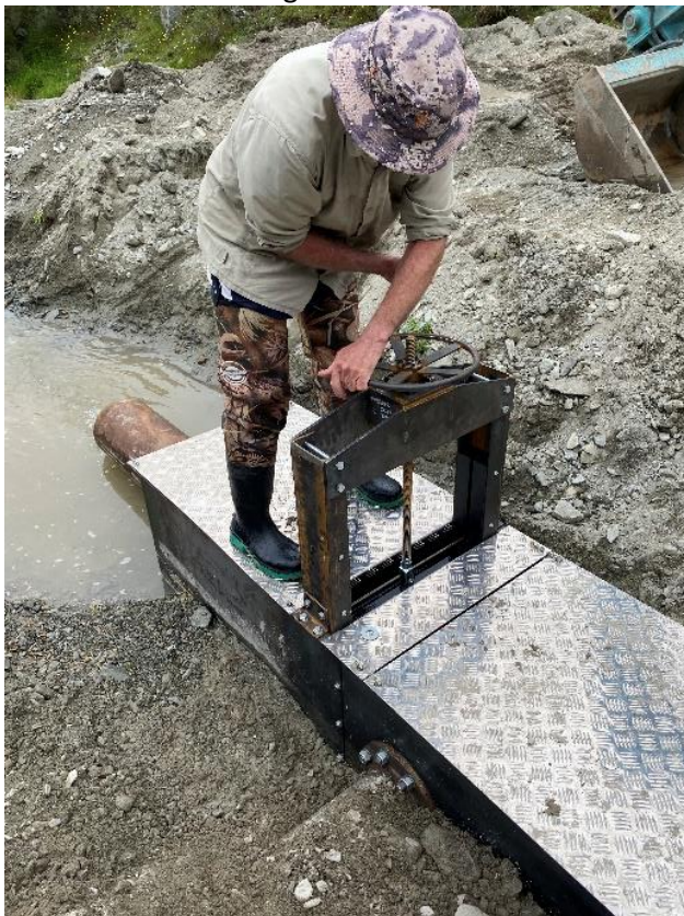
Photo 5. Flow control mechanism for irrigation intake and screen bypass (partially buried in gravel in central foreground), December 2021.
