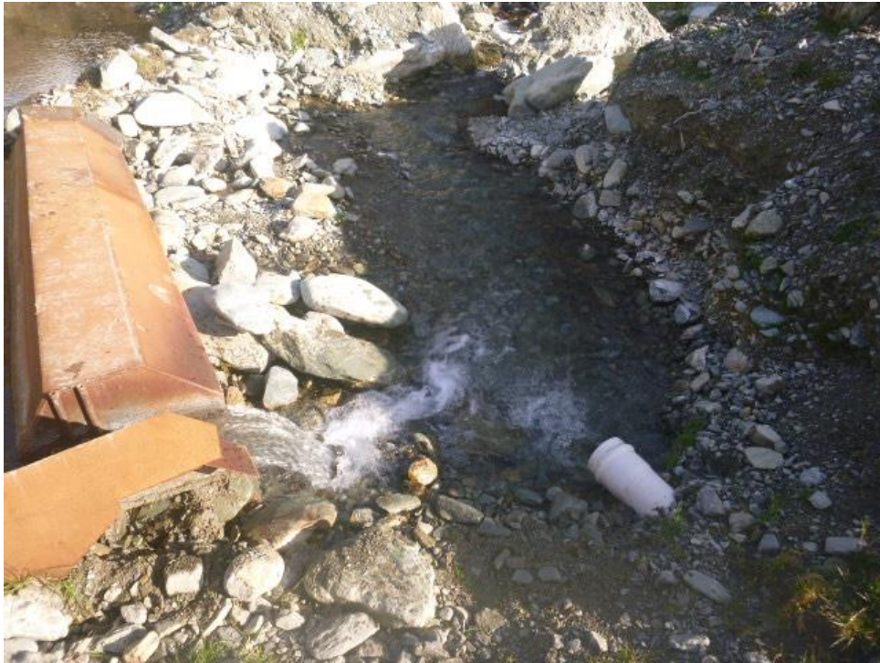
Photo 8. Fish screen bypass pipe (right) discharging to river return and upstream bypass (left) discharging from steel apron. February 2022.
