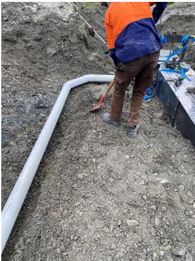
Photo 7. Screen bypass pipe prior to burial, December 2021.
