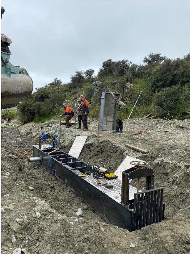
Photo 6. Fish screen placement. Piped screen bypass outlet on left side of fish screen, December 2021.
