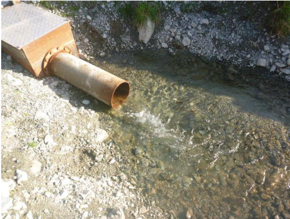
Photo 4. Outlet to irrigation from downstream end of fish screen, June 2021.
