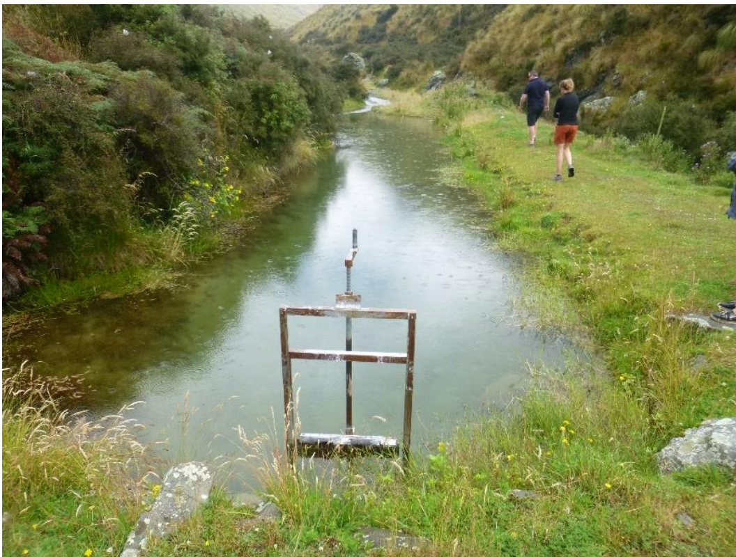
Figure 1 View upstream of intake channel from West Awakino River in the background and flow control gate regulating flow to irrigation head pond under Deemed Mining Permit conditions
