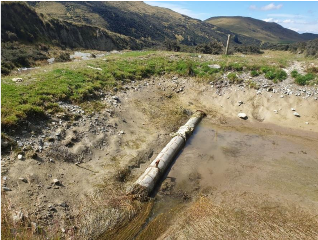
Figure 3 View downstream towards the irrigation take of drained irrigation head pond with perforated pipe fish screen on the bed under Deemed Mining Permit conditions
