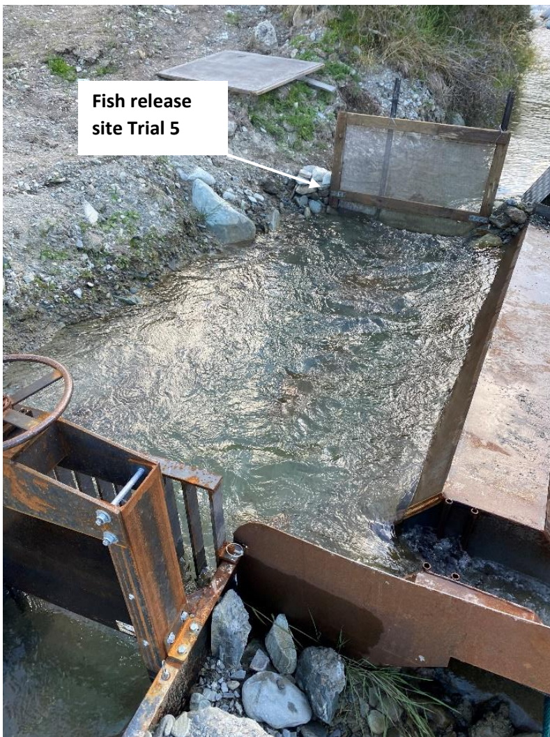
Figure 7 Screen intake on left with prefabricated steel base insert and temporary upstream screen to confine fish. upstream bypass exit at bottom right. February 22.
