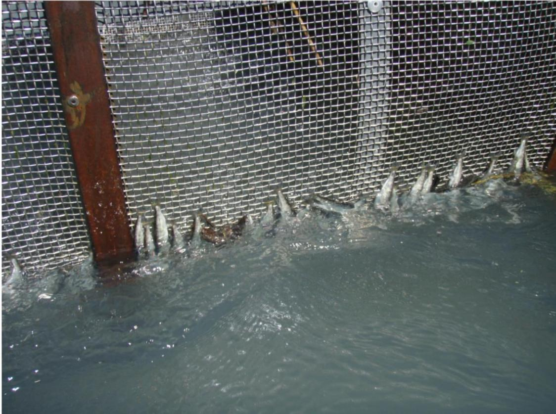
**Figure 10:** Chinook salmon trapped on the upstream side of a woven wire rotary drum screen. Photo credit: NIWA.
