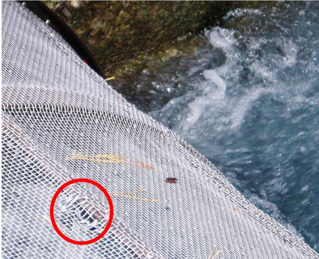
**Figure 15:** A rotating drum screen where gaps appearing over time is an issue with this screen type. Note, the red circle is highlighting an area where the mesh has been stretched resulting in larger gaps.
